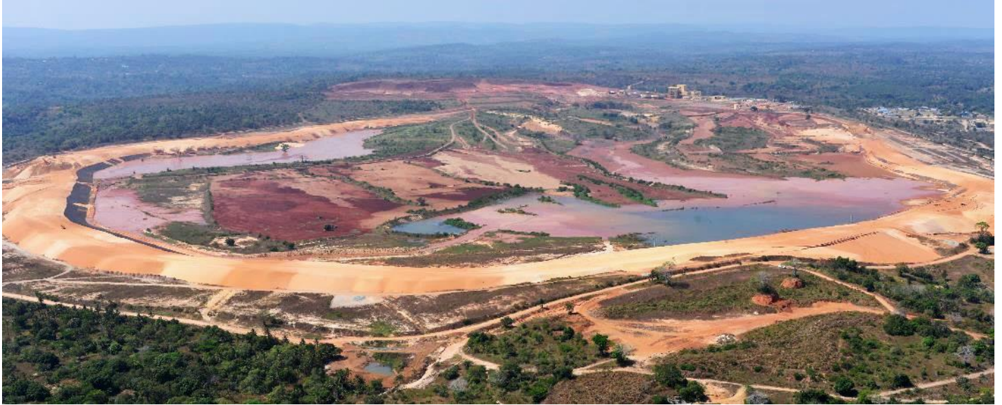
270 Hectare Tailings Storage Facility
